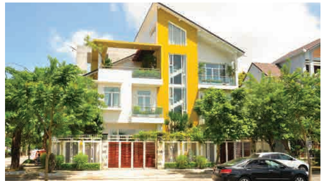
Villa at Ly Nhan Tong street, Danang
