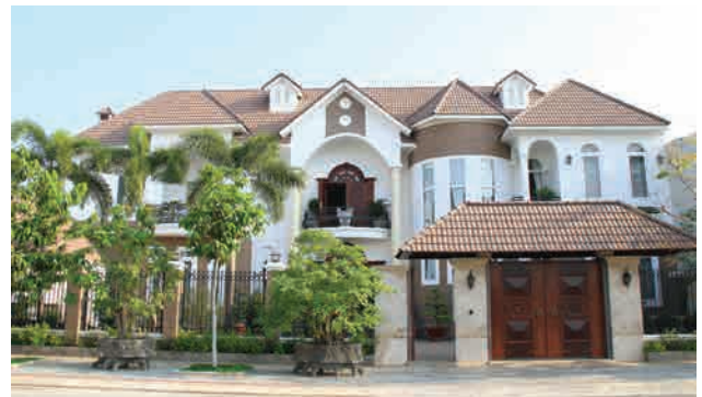
Block 1 – 2 – 3 – 4, Hung Vuong Residential District, Phu Thuy Ward, Phan Thiet City, Binh Thuan Province
