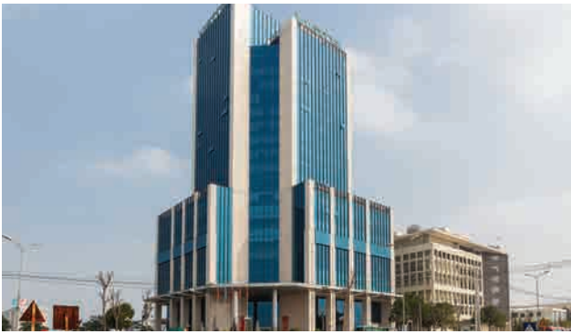
Viettel High-tech Building, Thang Long Boulevard, Thach That, Ha Noi
