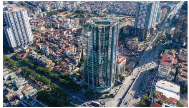
VP Bank Tower, 89 Lang Ha Str., Hanoi City
