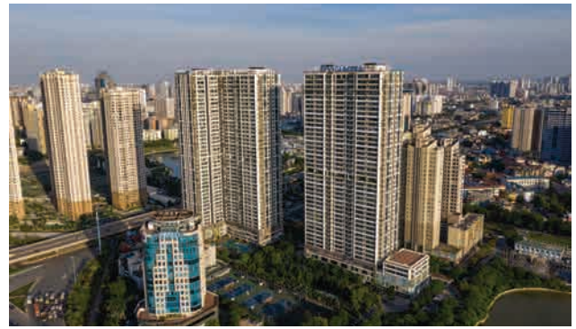
Viglacera Tower, Thang Long Number 1, No.1 Thang Long Avenue, Hanoi City
