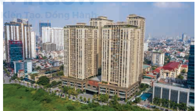
Homecity Apart (under construction), Trung Kinh, Cau Giay, Hanoi city
