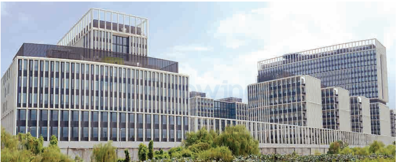
Ministry of Public Security Headquarters, Block B1, B3, B5, C, D & E - Pham Van Dong Str, Hanoi
