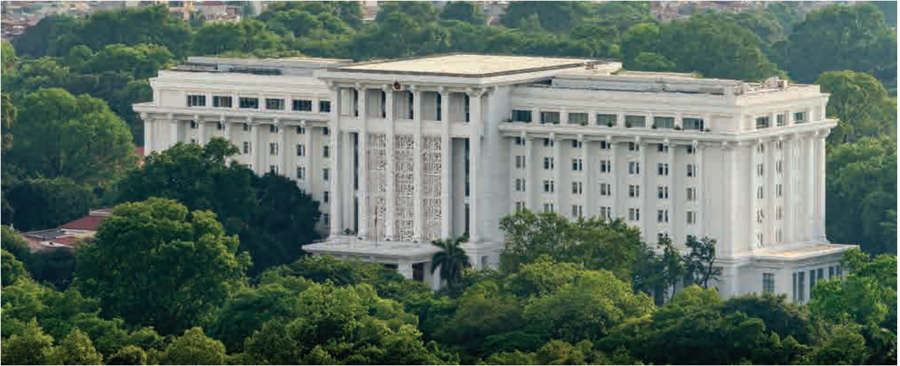
Government Office Building, No 01 Hoang Hoa Tham Str., Ba Dinh District, Hanoi.
