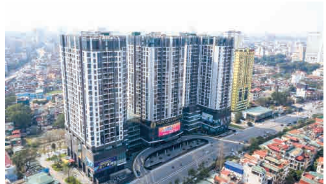
Sun Grand City Ancora Residence, 03 Luong Yen, Bach Dang Ward, Hai Ba Trung District, Hanoi City
